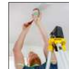
Plumb line - take a point from floor to ceiling
